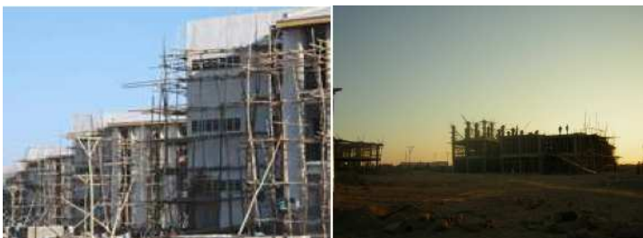
Status of Semera University during construction time, (2008-2009)
