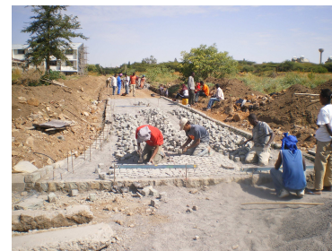
Cobblestone paved walkway in the premises of Adama University.
